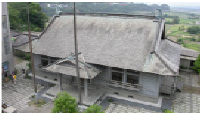
武德殿的「入母屋造」屋頂。 A hip-and-gable roof construction, called "irimoya-zukuri"
